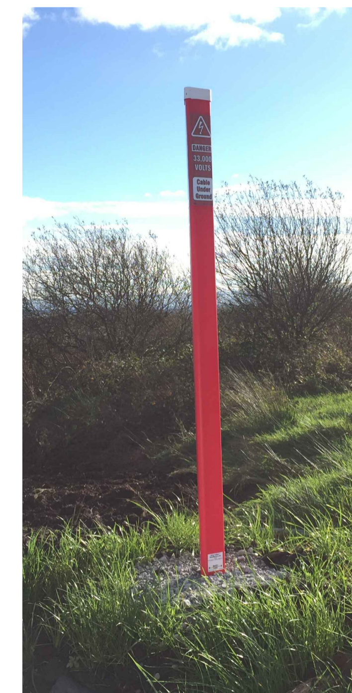
Typical Cable Marker Post
